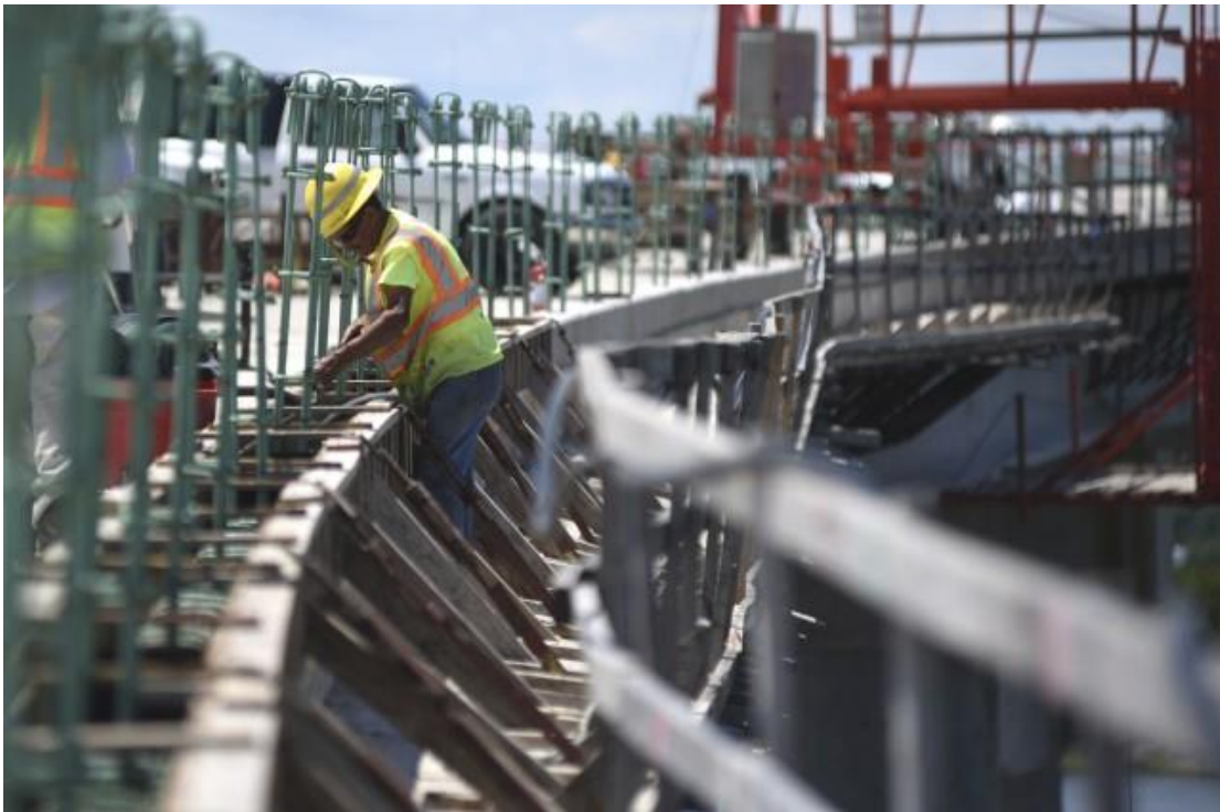
Figure 28. America's Infrastructure. Photo Credit: Matt Barnes. Source: Star News
